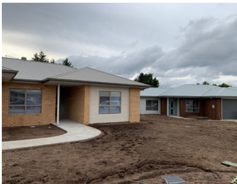
▲ The finished homes at Glenara Lakes Lifestyle Village in Launceston
